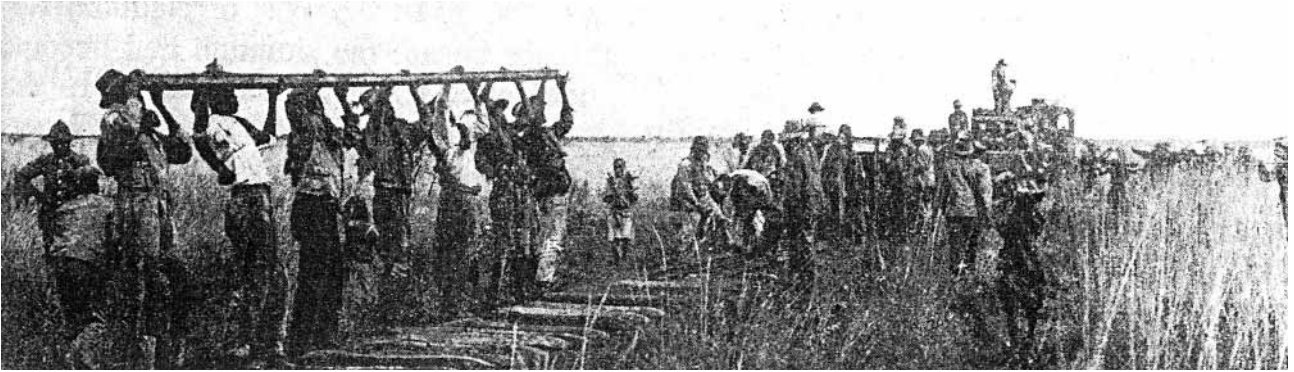
Construction of the Otavi Railway.
