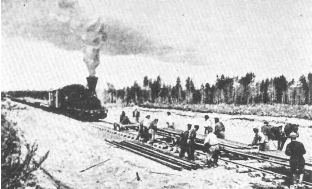
Russian workers laying the final lengths of track for the Trans-Siberian Railway.
