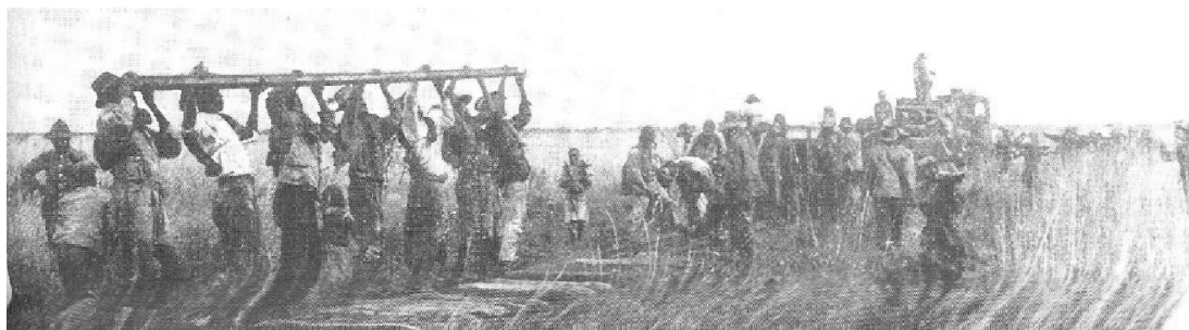
A photograph showing the construction of the Otavi Railway across Herero land in 1903.
